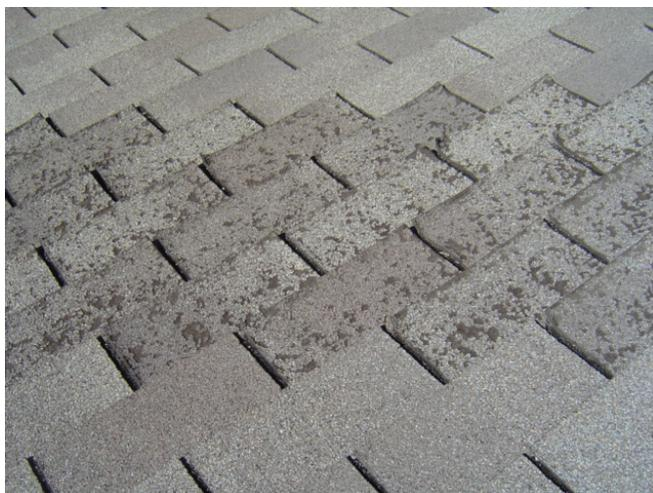
These shingles were the result of a manufacturing defect. Notice how a section of shingles is all that is damaged, this amounts to one bundle of shingles and is commonly installed in the manner shown.
